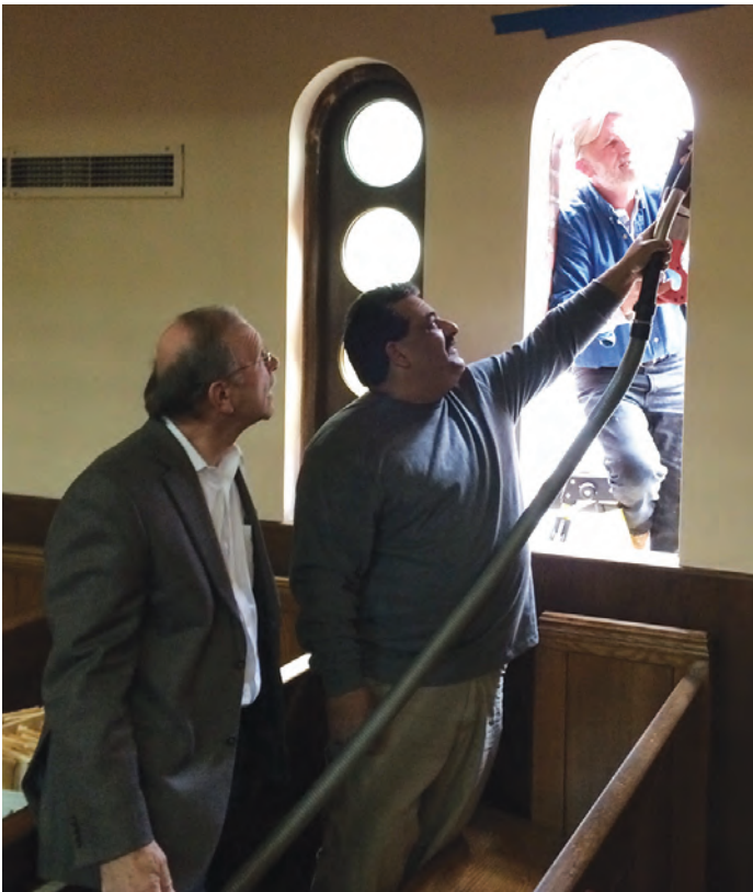
Tony & Richie installing replacement window as Nick Aivalis looks on (Dec 1)
