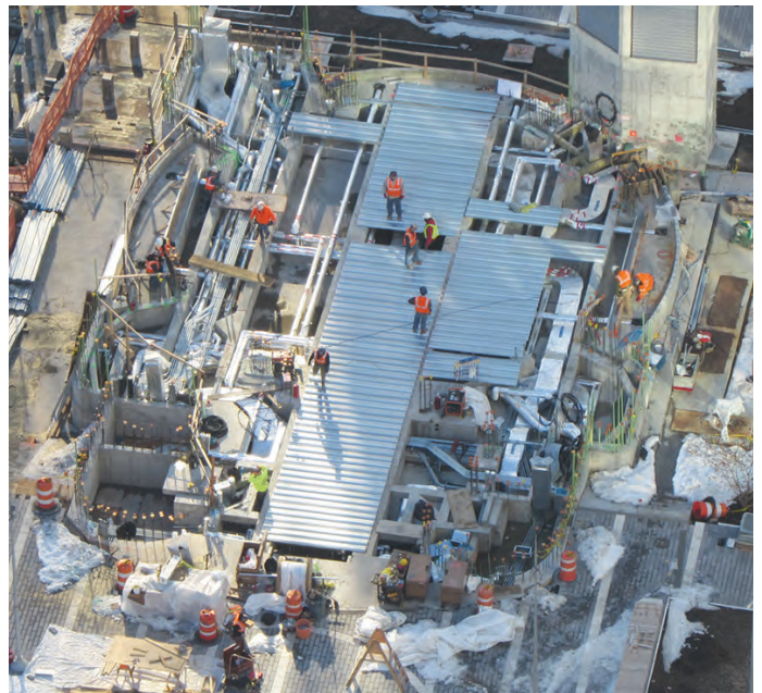
Aerial photo of metal deck being installed for St. Nicholas National Shrine at Ground Zero (Feb 2)
