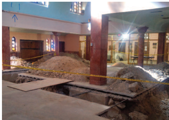
Removal of old air ducts took place throughout the month of August.
