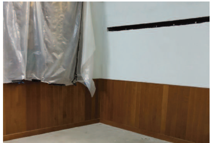
wainscoting completion
