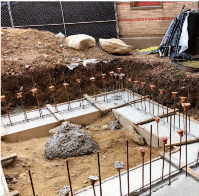
New concrete footings are poured at the rear entrance near the parking lot. (9-25-18)
