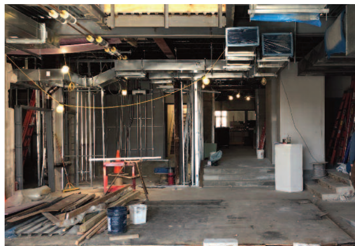
HVAC ductwork installation is well underway in the new rear entrance. (March 27)
